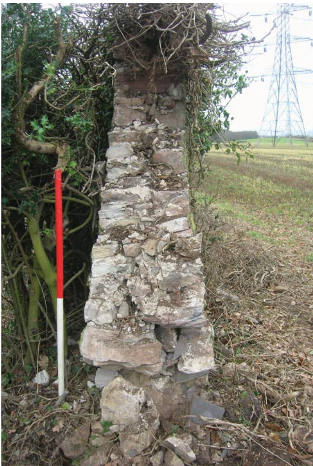
Illus 9.5 (left) Section through the western perimeter boundary wall showing double skin with rubble core
