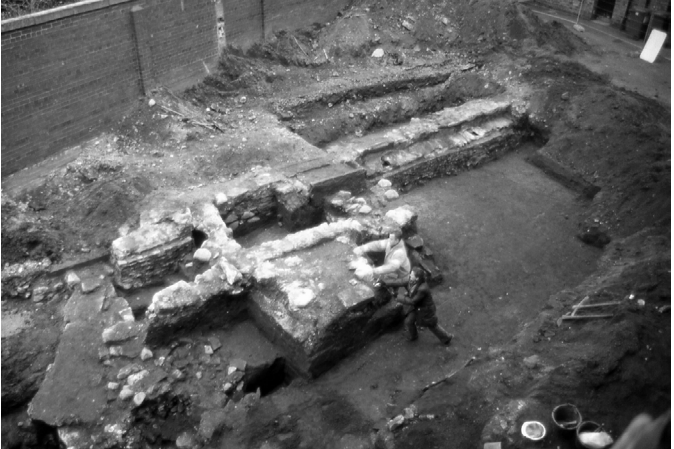
Illus 8 The foundations during excavation
