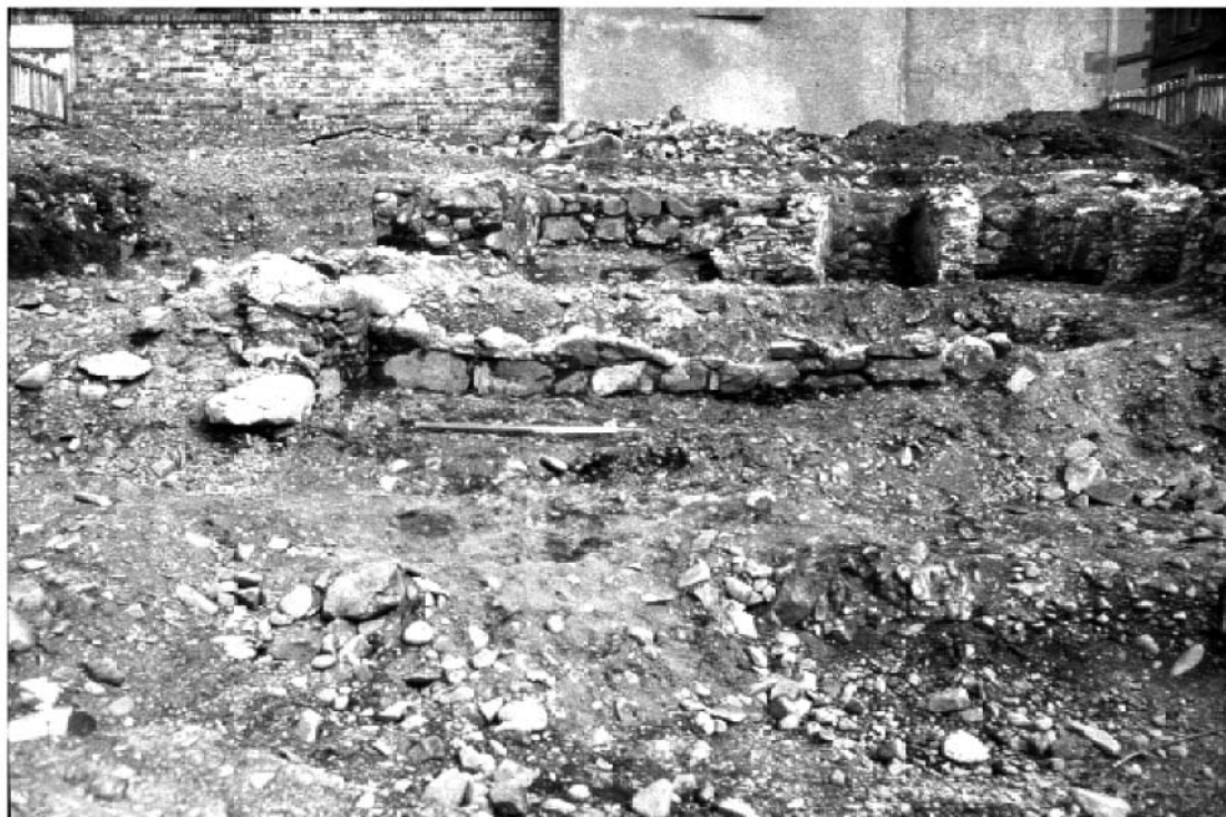
Illus 32 Bridgewater, Peebles, view of Building 1 from west, with cross-wall in centre and east wall in background
