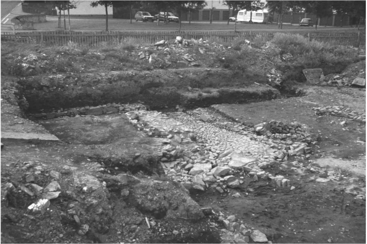
Illus 40 Bridgegate, Peebles, view of Building 4 from south-east (before extension of excavation to reveal stone pits)
